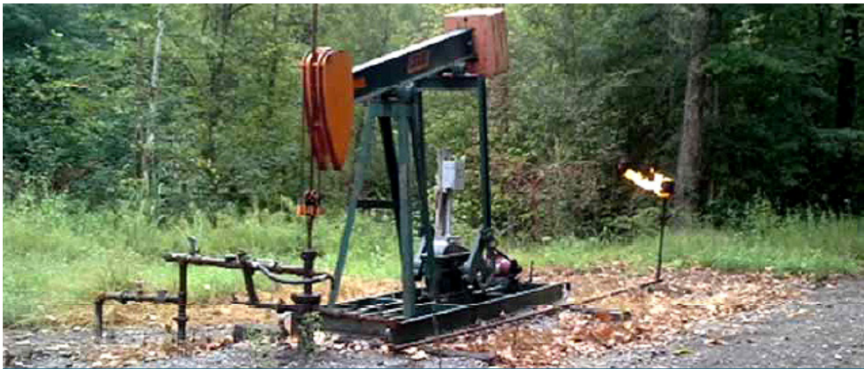
FIGURE 4. Permanent casinghead gas flare on a producing stripper oil well in Hopkins County, Kentucky. Photo courtesy of Marvin Combs, Kentucky Division of Oil & Gas (Source) 4
